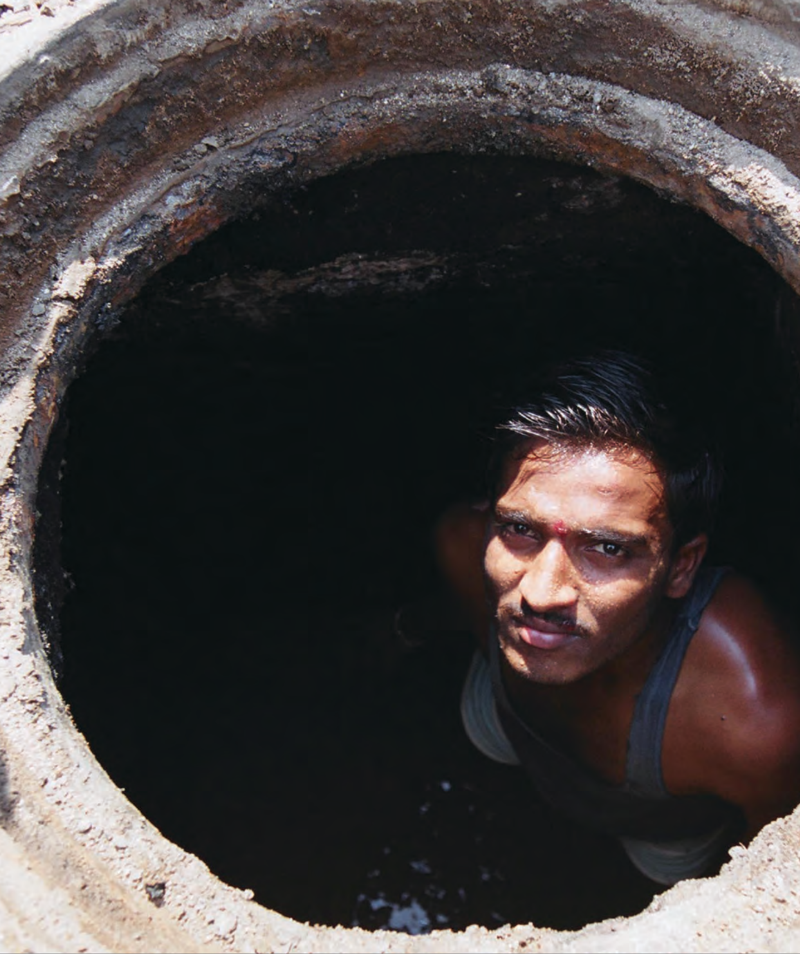
Prakash, sewage worker in Hyderabad, works in the sewer without any protection—no gloves, no suit, no boots. He uses his hands and feet to scrape and clean out the sewage pipes. India, M. Crozet, 2002. © ILO. Used with permission. Permission required for reuse.
